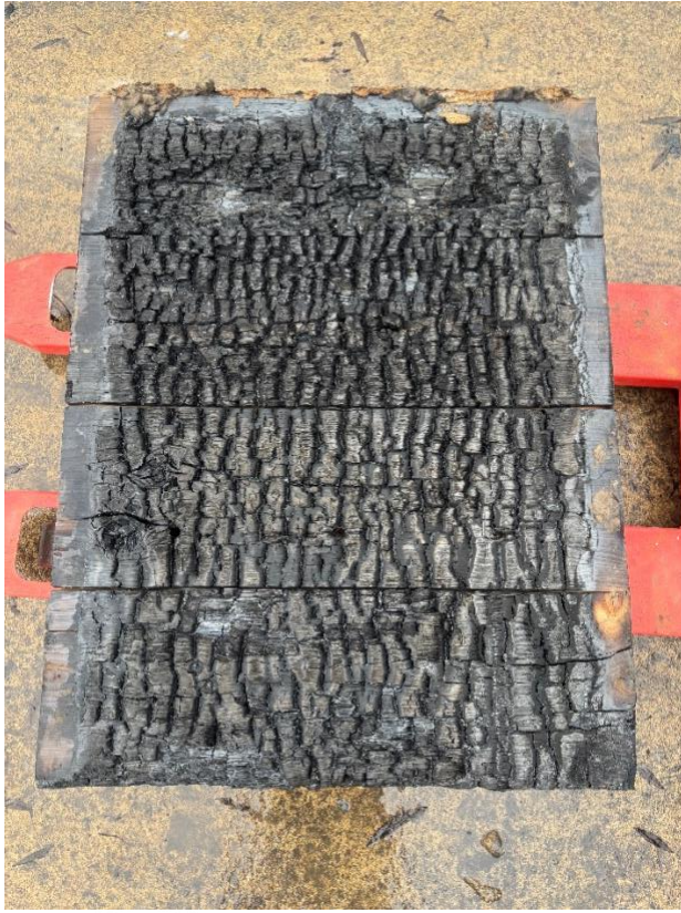
Figure 22 Ceiling panel post fire
