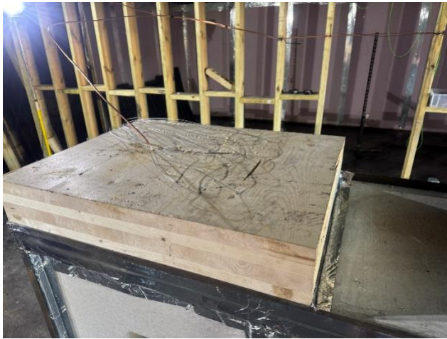
Figure 13 CLT ceiling panel
