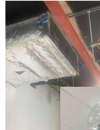
Sealed ductwork to prevent dust ingress
