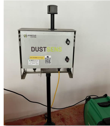
Dust monitor on live floor
