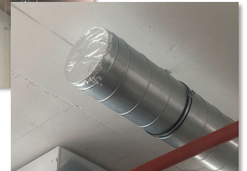
Sealed ductwork to prevent dust ingress
