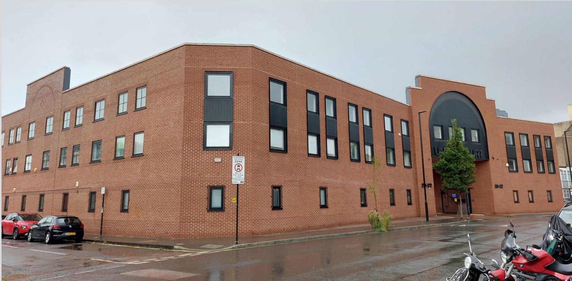
Keim Restauro Lasur colour wash after completion
