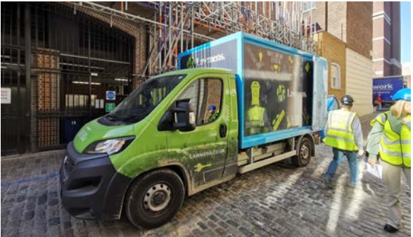
Removal of reuse material via electric vans
