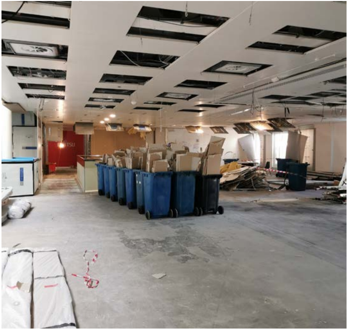
Soft strip out of ceilings
