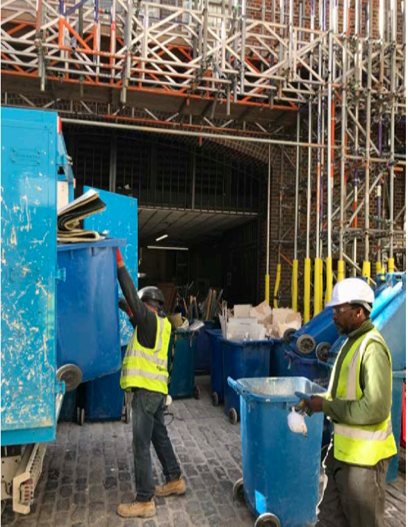
Removal of reuse material to be sorted
