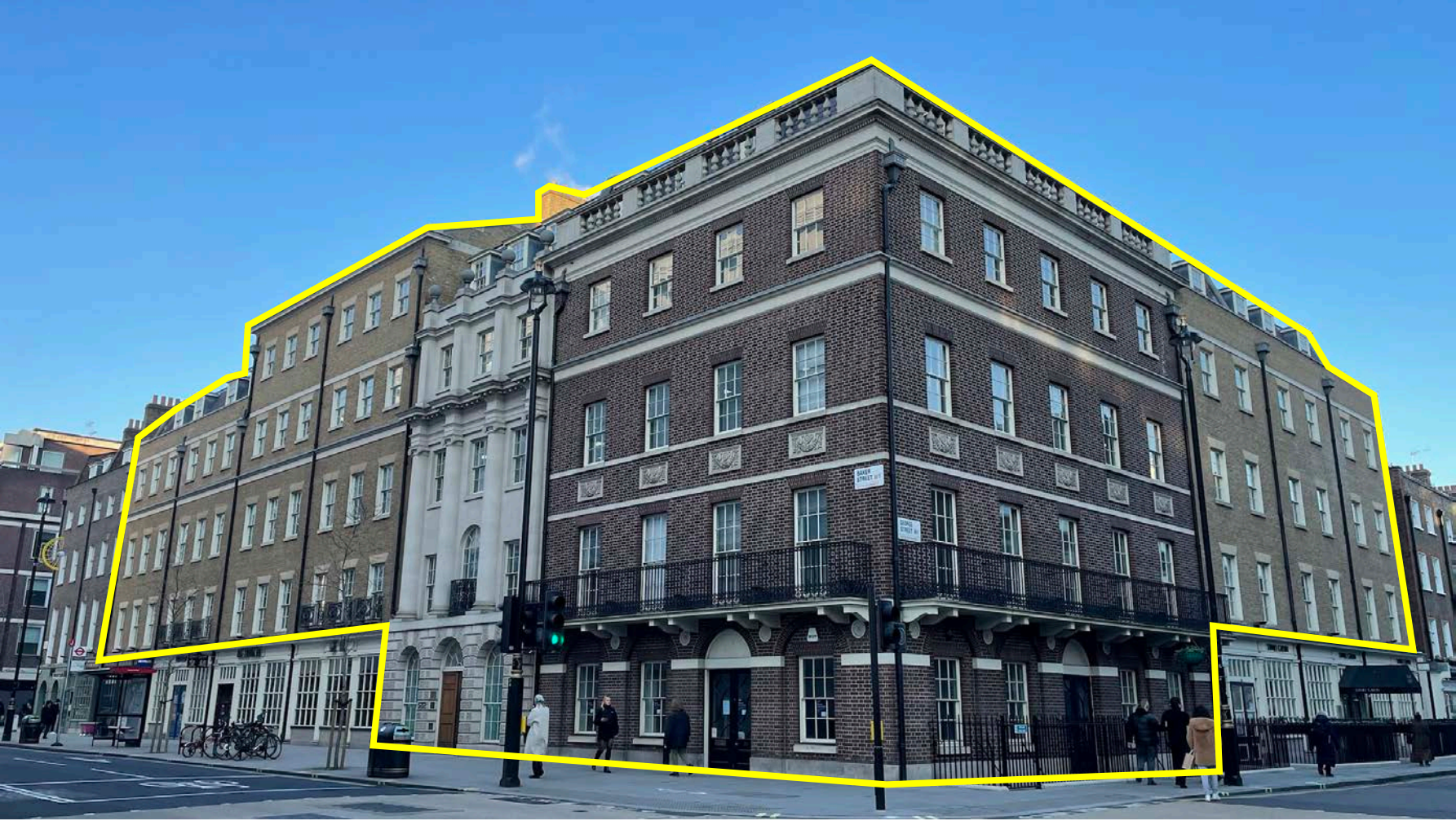
Existing External View of Office Building
