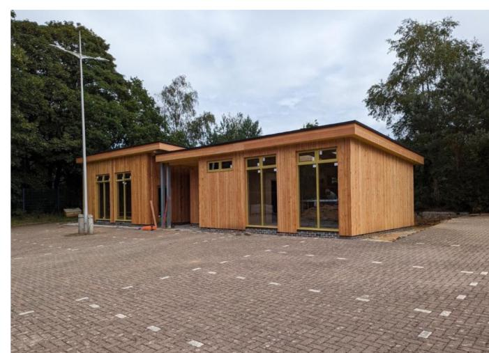
ADEPT, is a bio-based construction solution designed for adaptation, disassembly and re-use.
