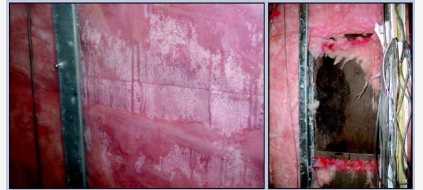
Water vapor diffusing inward during summer conditions in a cold climate (Waterloo, Canada) condensing on a low-permeance vapor barrier. The resulting damage is shown at right.
