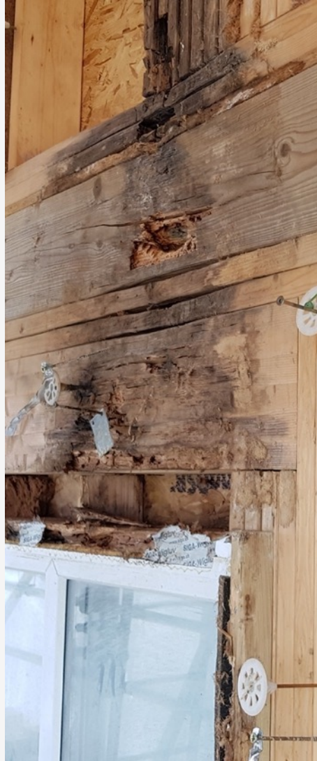
Water vapor diffusing inward during summer conditions in a cold climate (Waterloo, Canada) condensing on a low-permeance vapor barrier. The resulting damage is shown at right.
