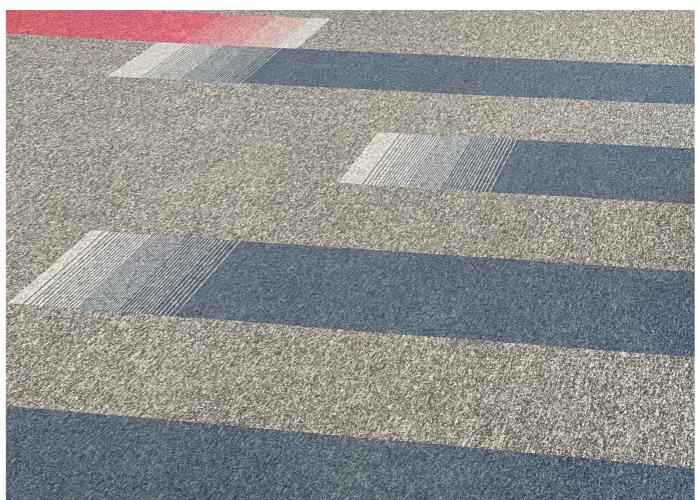
Floor coverings installed using adhesives can be difficult to reuse or recycle on uplift, due to contamination.
