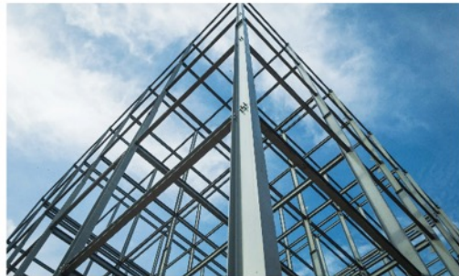
Unsuccessful steel reuse case study
