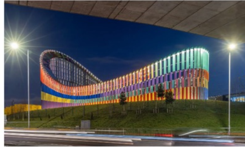
Brent Cross Town Primary Substation
