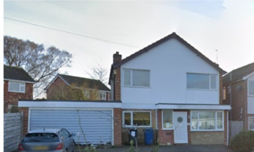
Steel reuse domestic refurbishment project
