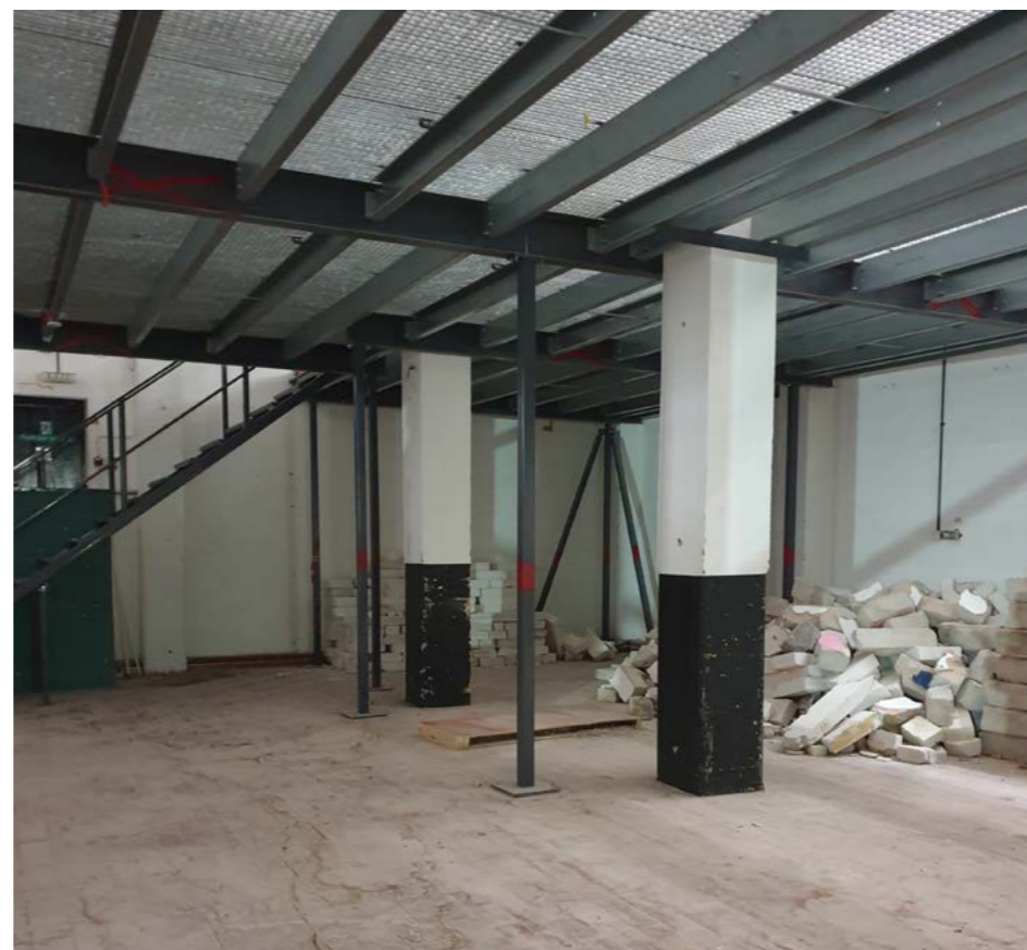
Steel beams and columns forming mezzanine
