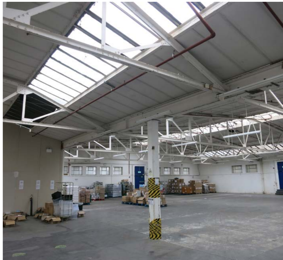
Steel trusses
