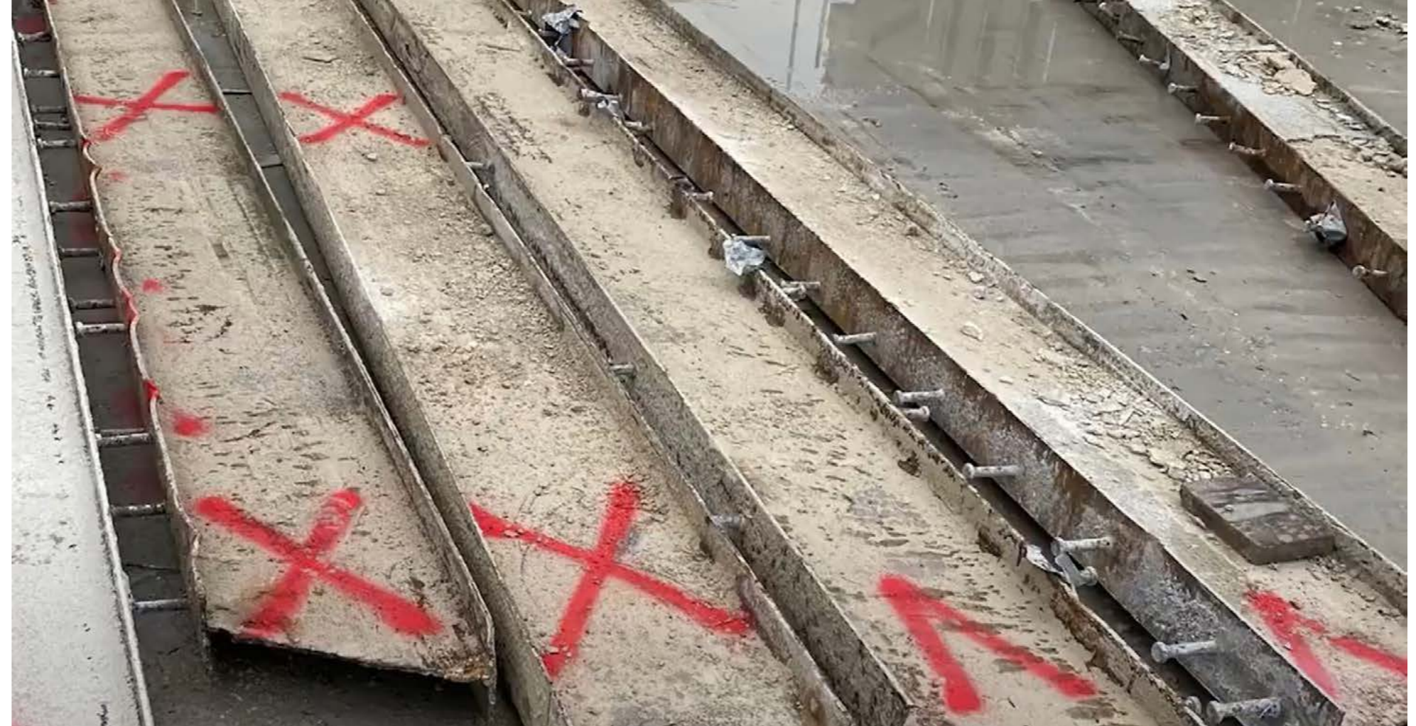
Extracted Steels from One Broadgate (Cantillon)
