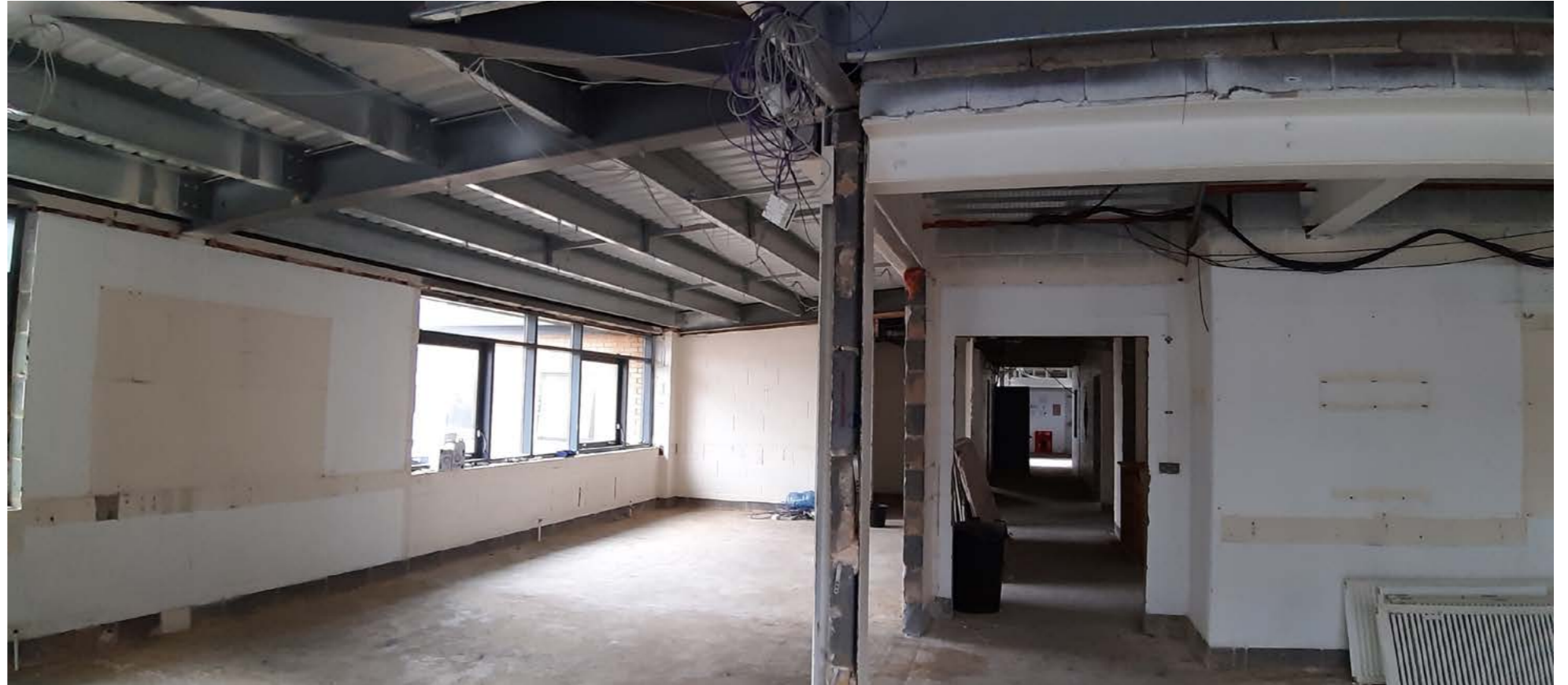
Compositely designed steelwork
