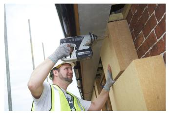
Installation of external woodfibre insulation. (Houlston Manor, Shropshire. Image courtesy of Lime Green Products)
