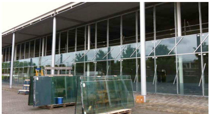
Dismantled façade to be transported to 9 Cambridge Avenue
