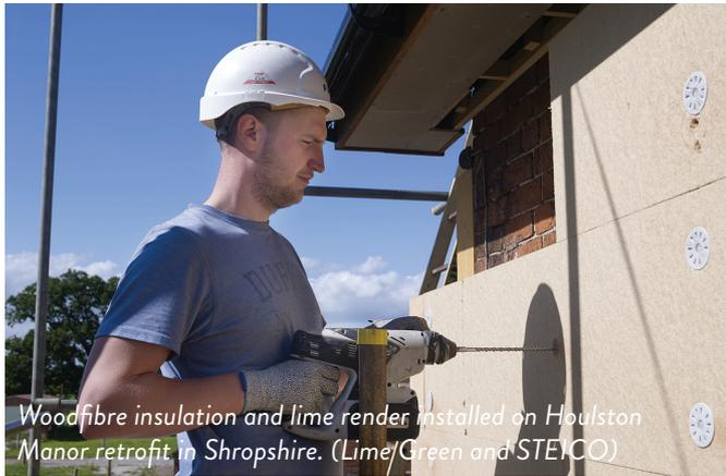
Woodfibre insulation and lime render installed on Houlston Manor retrofit in Shropshire. (Lime/Green and STEICO)
